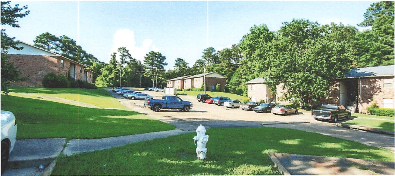
View at center of site to north
