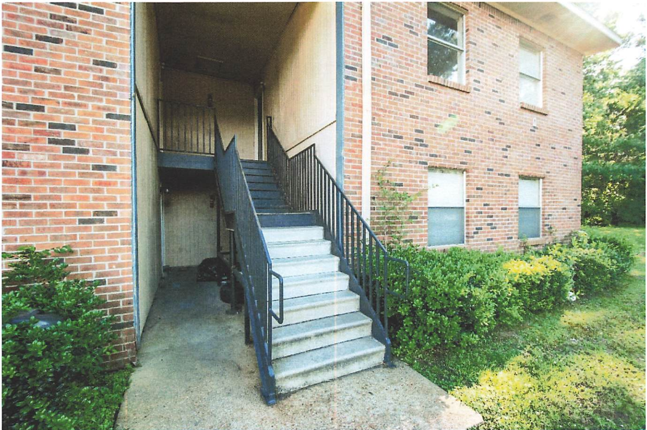
Typical Building Stair
