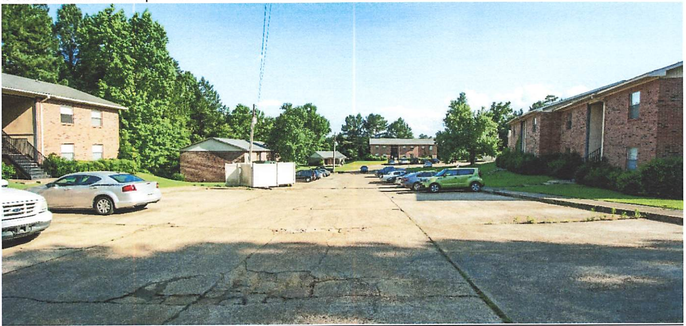
Main site road view to south
