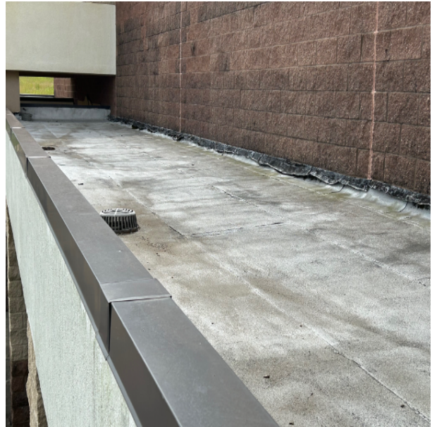
Overview of roof
