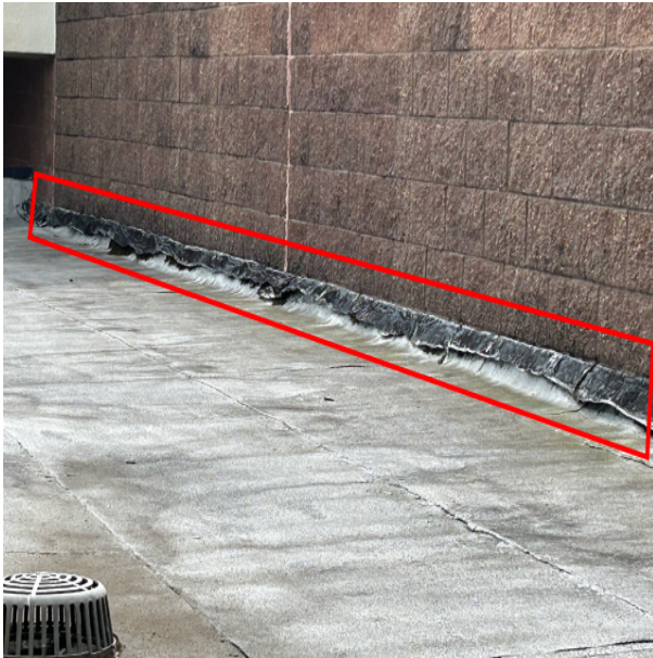
Area of Work
