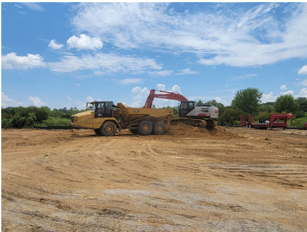
Loading Off Road Haul Truck from Stockpiled Borrow
