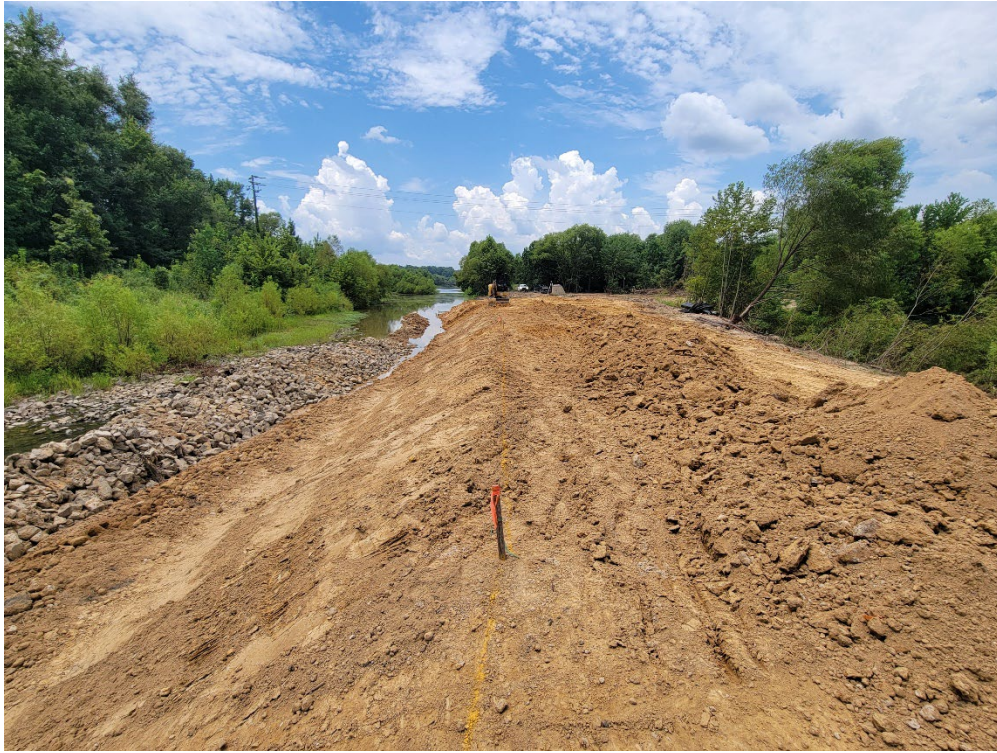
Starting to Armor Channel Embankment
