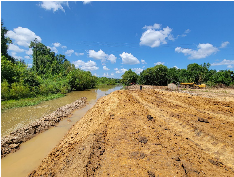
Pipe Has Been Encapsulated with Crushed Stone; Rough Grading Channel Embankment
