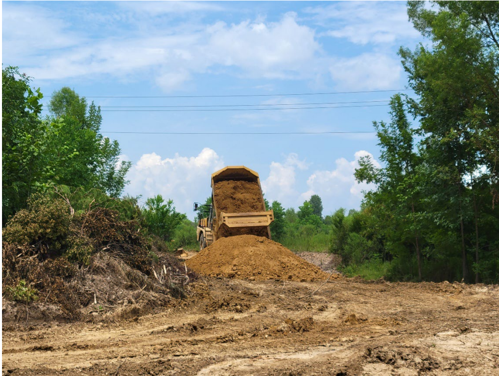
Off Road Haul Truck Transferring Borrow Material to Site
