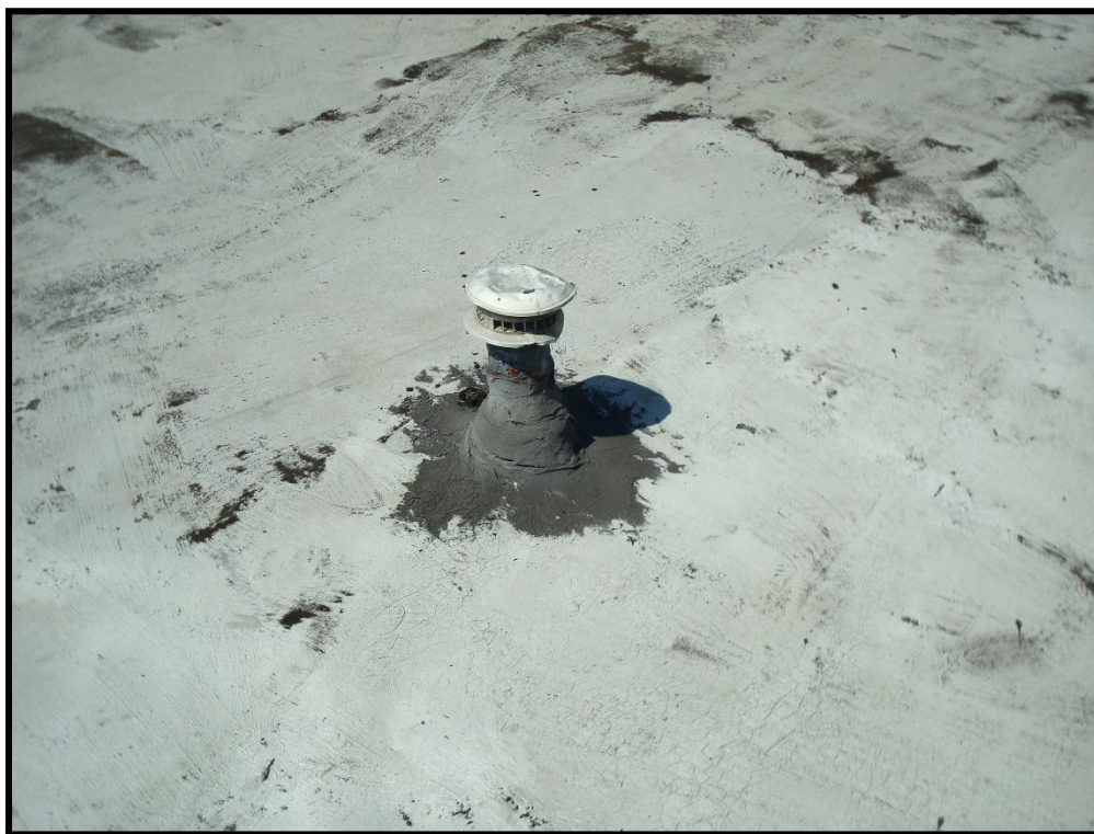
Penetration Flashing (HA) (756-04)
