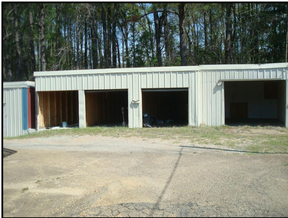
Metal Storage Building at 756 West Government Street
