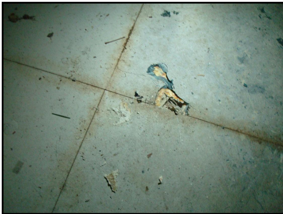
2 nd Layer Linoleum under Floor Tile (HA) (714-06)
