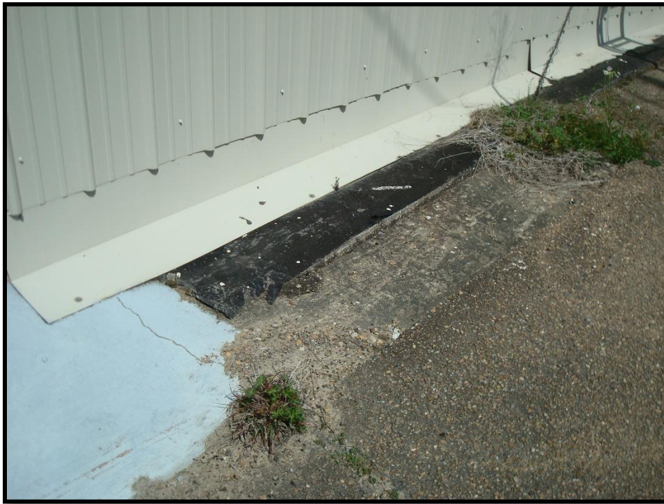
Black Felt on Concrete Pad (HA) (756-12)
