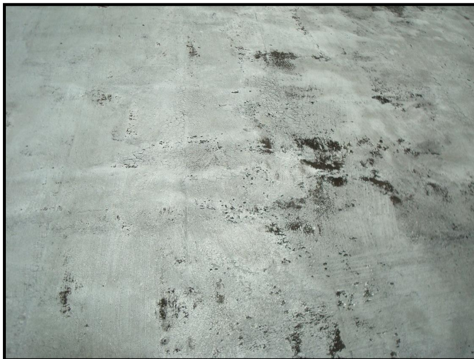
Roof Core (HA) (756-05)
